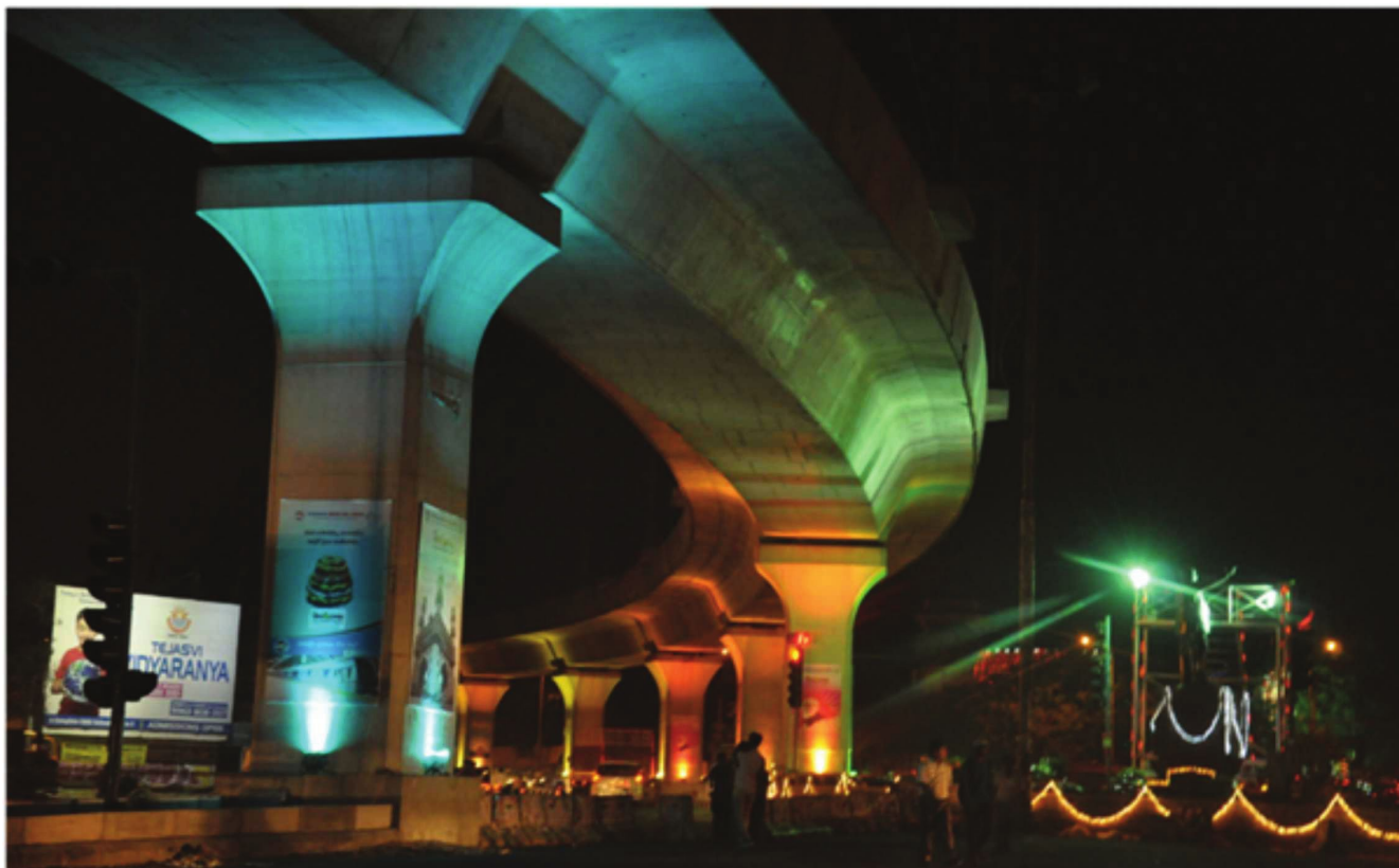
Hyderabad Metro Rail Project
