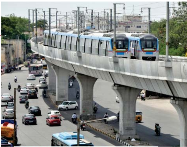
Metro Rail elevated viaduct – with two trains
