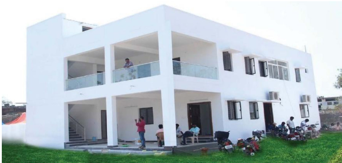
MLA Office- cum -Residence, Parkal
