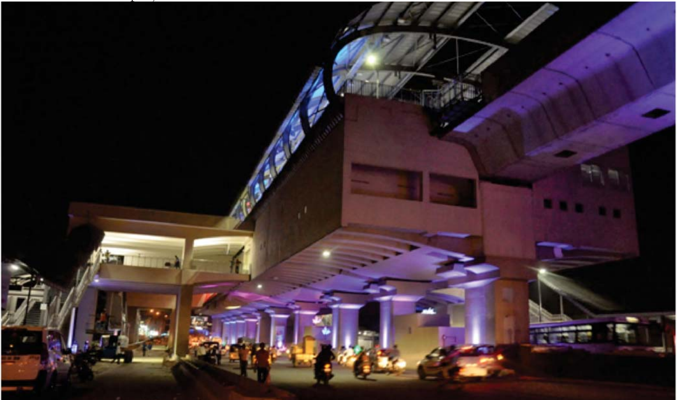
Hyderabad Metro Rail Project
